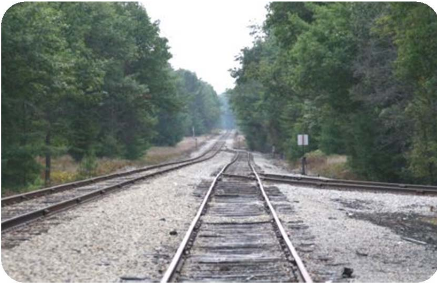
Figure 19: A view looking south at the existing railway line in Walton
