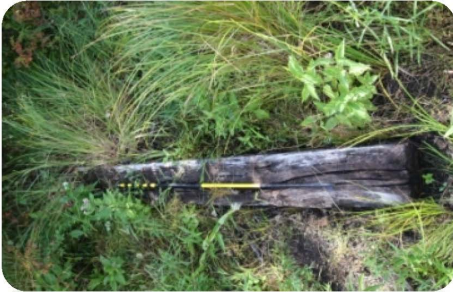
Figure 16: Examining a railroad tie at the shoreline 4 Ft. scale
